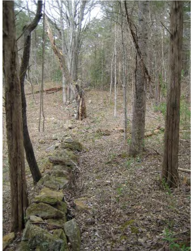
Figure 127. Sediment has filled upper side of wall (on right). Note the dead red maple that grew on the wall.
