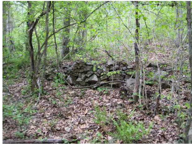
Figure 109. Rock wall built to support an old road to Hydraulic Mills.
