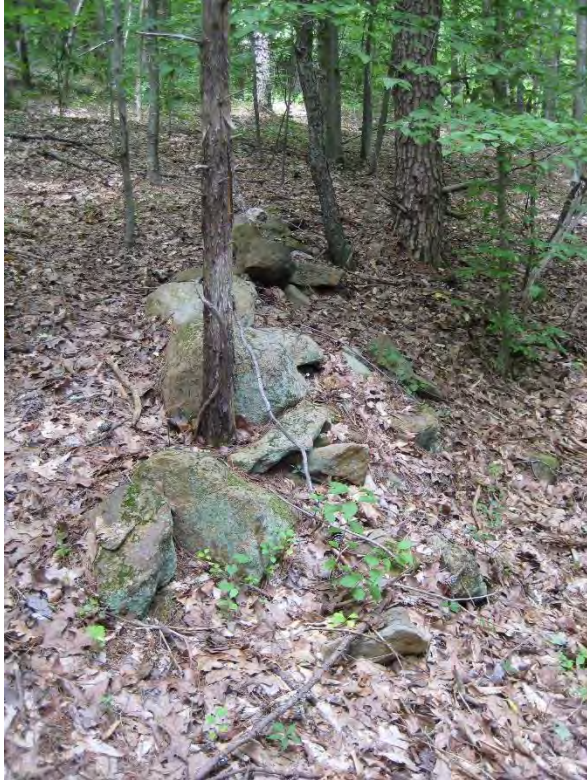
Figure 116. Rock wall that once supported an old road.
