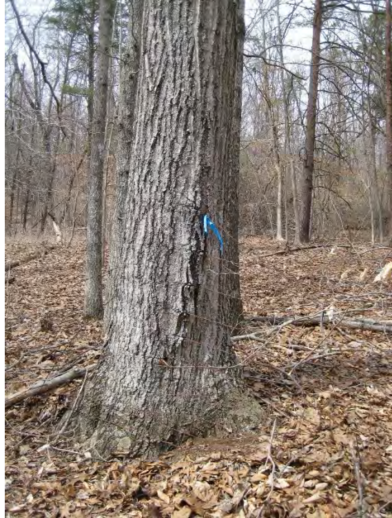
Figure 96. Fence line tree with embedded barbed wire that was nailed to it when it was a small tree.
