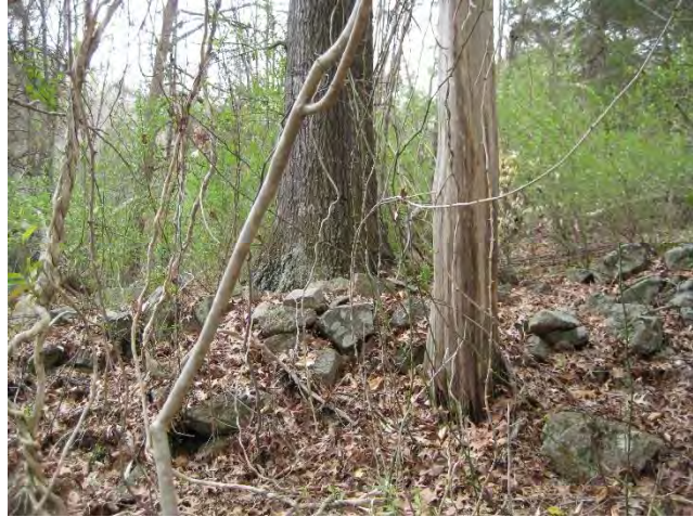
Figure 130. Short section of rock wall on east end of fence line.
