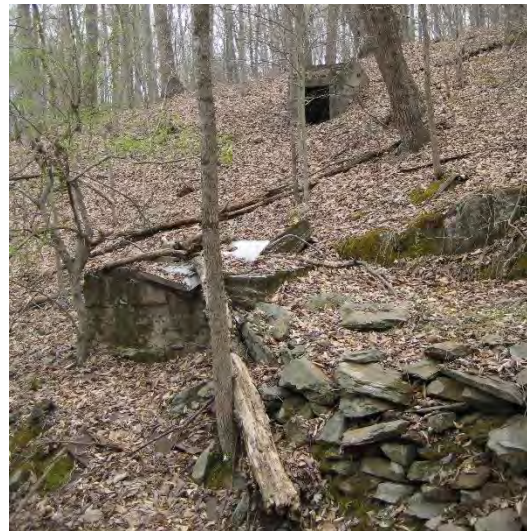
Figure 87. Pump house (above) and storage box (below).
